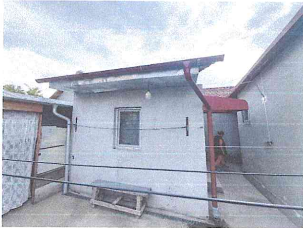
Constructia C2 -Anexa
